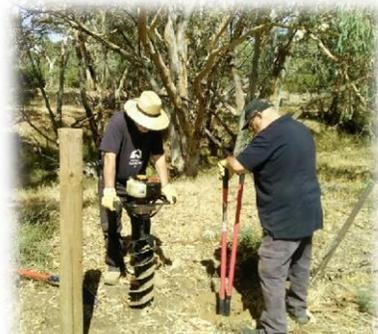
Fig 3 drilling holes for posts
