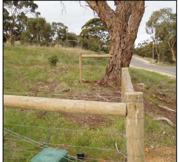
A simple strut arrangement that allows a fence to deviate a short distance around a tree. Wires are not attached directly to the tree, thus minimising potential damage to the tree.
